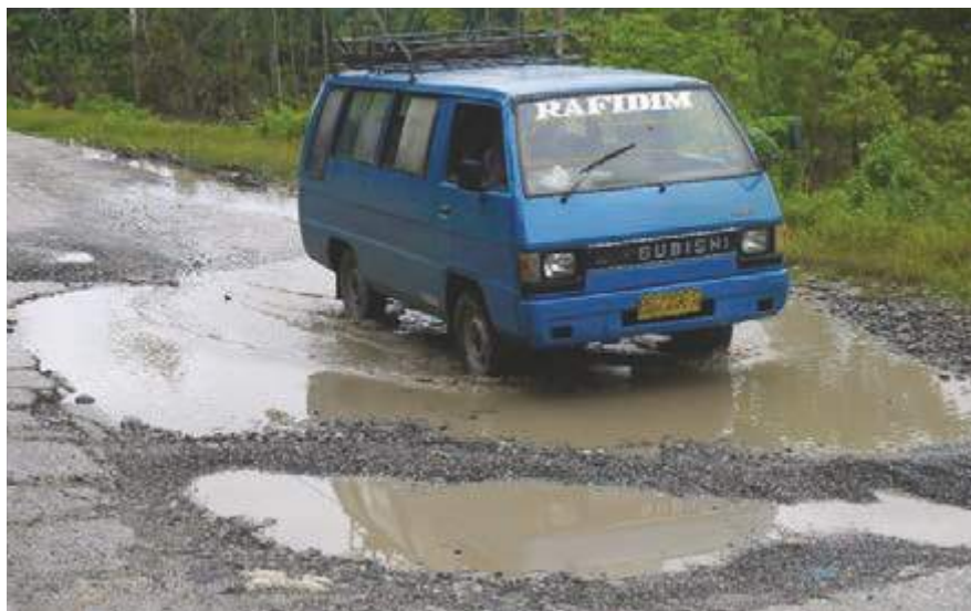
Figure 2: Potholes in tropical roads (photo © Mohammed Alamgir)
