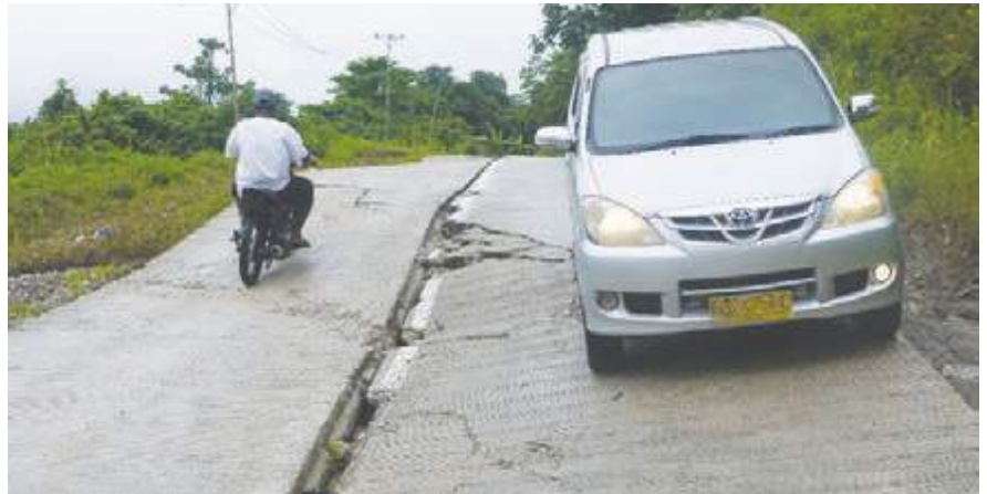
Figure 3: Slumping in tropical roads (photo © Mohammed Alamgir)
